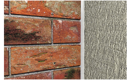
Vertical construction joint application
