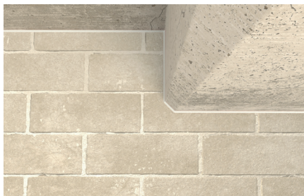
Construction joint application
