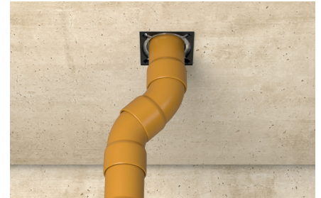
Installed pipe through FCID Plus device
