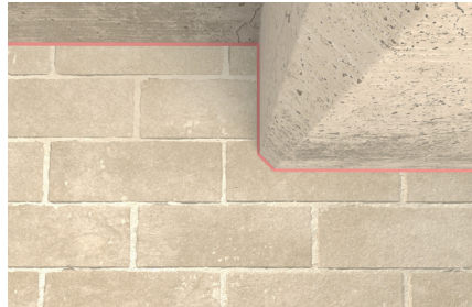
Construction joint application
