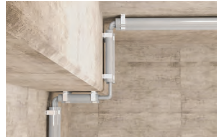
Fixing plastic insulating conduits
