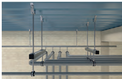
Suspended pipes on trapezoid roof
