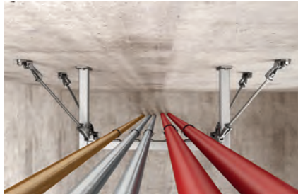
Bracing of frame construction with threaded rods
