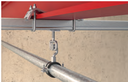
Channel to steelbeam
