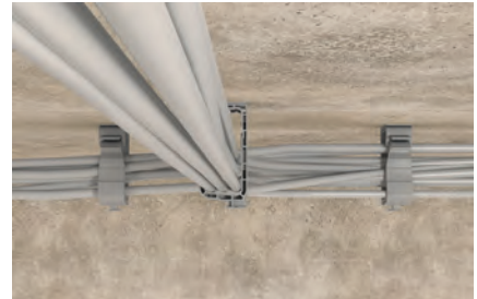
Fixing cable bundles
