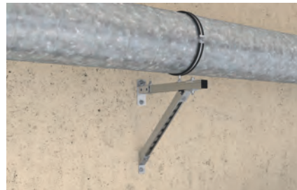
Spiral airduct on cantilever
