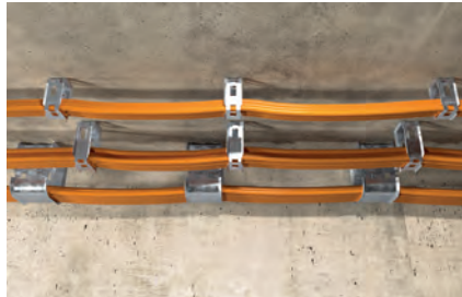
Cable fixing to the ceiling
