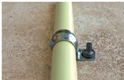
Fixing armoured conduits
