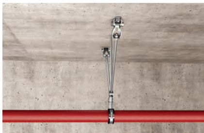
Bracing of pipeline with threaded rods
