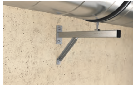
Ventilating pipe fixing at the wall
