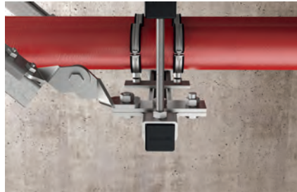
Bracing of channel construction
