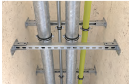
Pipe installation in escape route
