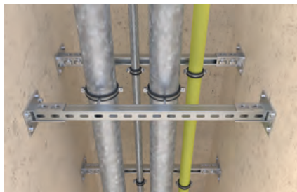
Pipe installation in escape route
