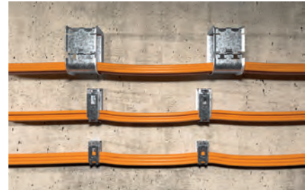
Cable fixing to the wall
