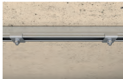
Channel installation at wall
