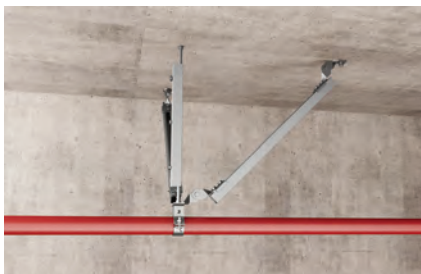
Pipe installation with seismic pipe clamp
