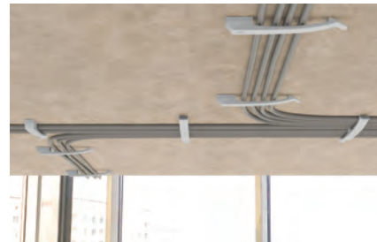
Fixing cable harnesses
