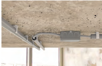
Fixing plastic insulating conduits
