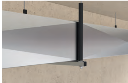
Air duct fixing with channel
