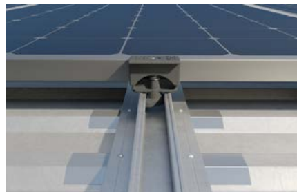
Roof with trapezoidal metal sheets covering
