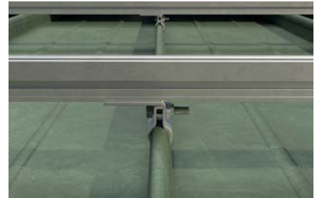
Pitched roof with rounded standing seam covering
