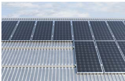
Roof with trapezoidal metal sheets covering
