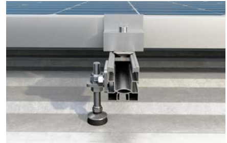
Roof with trapezoidal metal sheet covering
