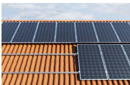
Pitched roof with barrel tiles
