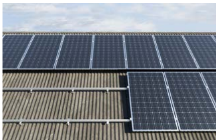
Pitched roof with corrugated sheets covering
