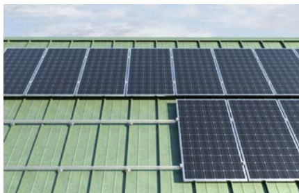
Pitched roof with flat standing seam covering
