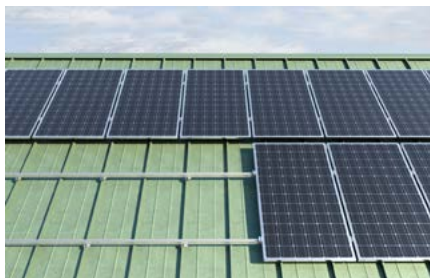
Pitched roof with standing seam covering
